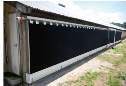
Figure 17.11 Cooling pads at air inlets in a tunnel house. The cooling pads reduce air temperatures experienced by the birds. (Photo courtesy of Michael Czarick, University of Georgia Cooperative Extension Service)
