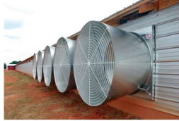
Figure 17.10 Exhaust fans moving air through a tunnel house. (Photo courtesy of Michael Czarick, University of Georgia Cooperative Extension Service)
